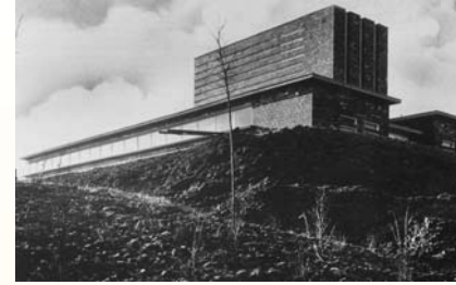
Königsberg (Kaliningrad/Russia), cemetery building erected in 1927, destroyed in 1938
